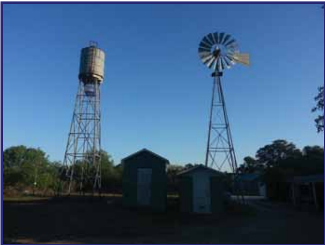
The Windmill and the Storage Tank
